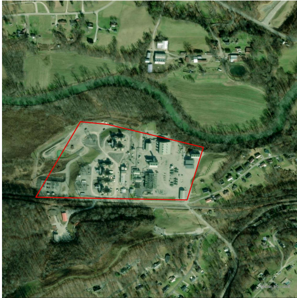
(c) Ceredo Power Plant (Gas) in Ceredo, USA
